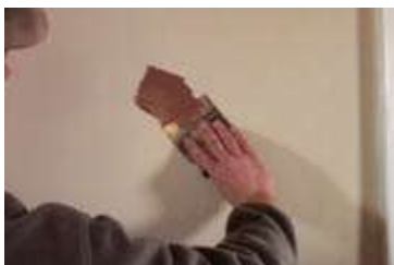
Photo 4: "X-ing" over the plaster, removing the excess.
