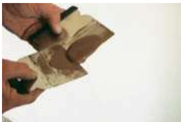
Photo 6: The plaster on one blade (the hawk) with the second blade positioned perpendicular to the hawk.
