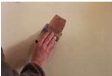
Photo 5: Using thin applications before slowly building up the thickness.
